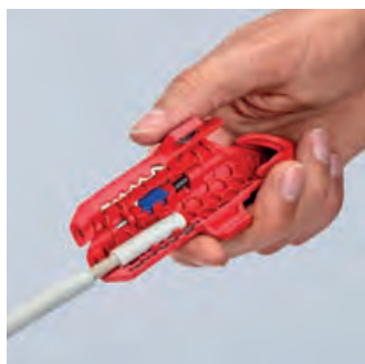
Stripping of a NYM cable
